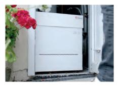
Watch the video to take a closer look at the key stages for the installation of Kensa Shoebox ground source heat pumps into individual flats in tower blocks, connected to shared ground loop array boreholes.
