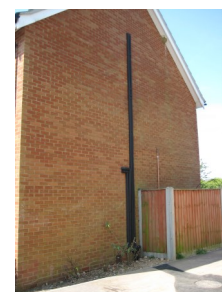
Gable end pipework feeding the two storey flats (to be cased).
