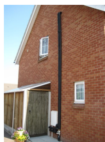
Pipework (to be cased) feeds through the wall and loft into both properties.
