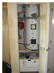
The Shoebox and new hot water cylinder in the airing cupboard.
